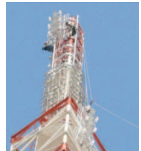
Installation of new integrated DAB+ and DTV Panels
