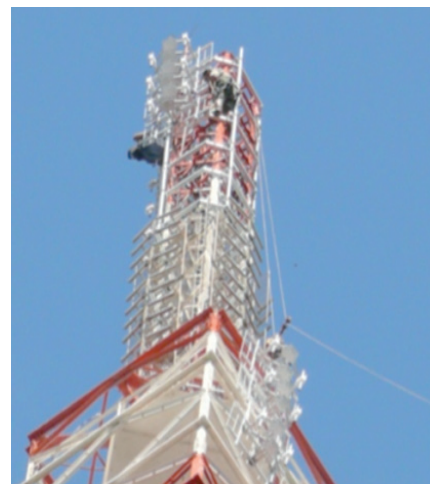
Installation of new integrated DAB+ and DTV Panels
