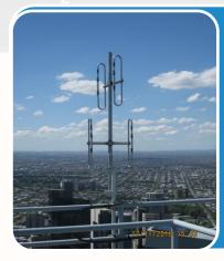
Low powered on channel repeaters (10 W – 1000 W ERP) to provide enhanced coverage where needed.
