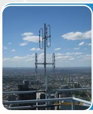
Low powered on channel repeaters (10 W – 1000 W ERP) to provide enhanced coverage where needed.
